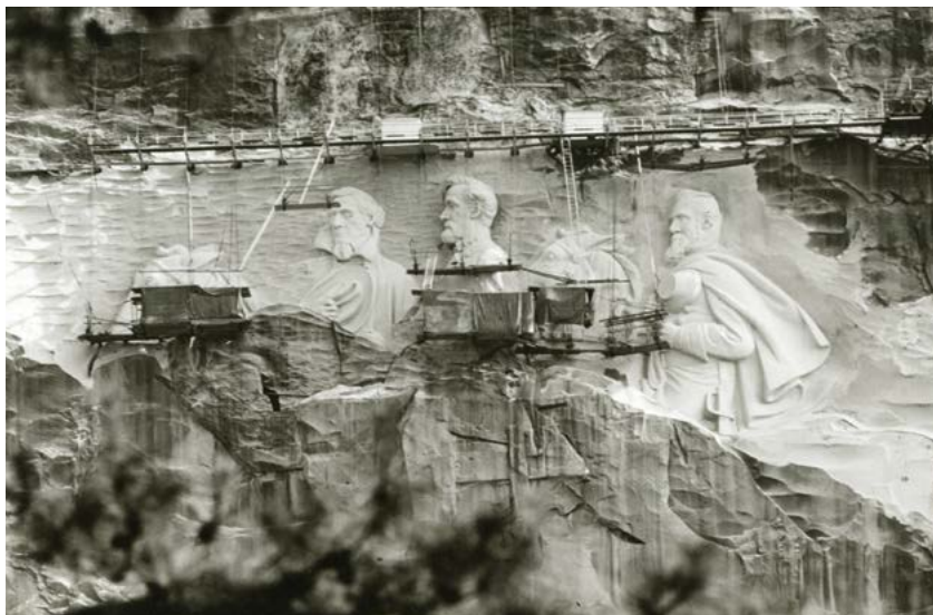
View of the 20th century carving at Stone Mountain in progress, undated. Kenan Research Center at Atlanta History Center
