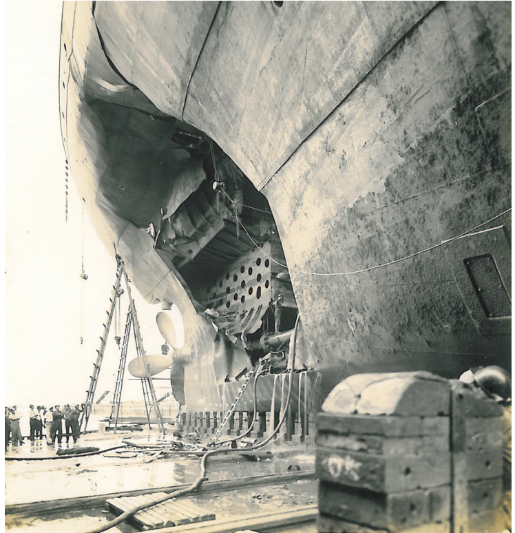
Torpedo damage on SS Oklahoma , attacked by U-123 on April 8, 1942.
